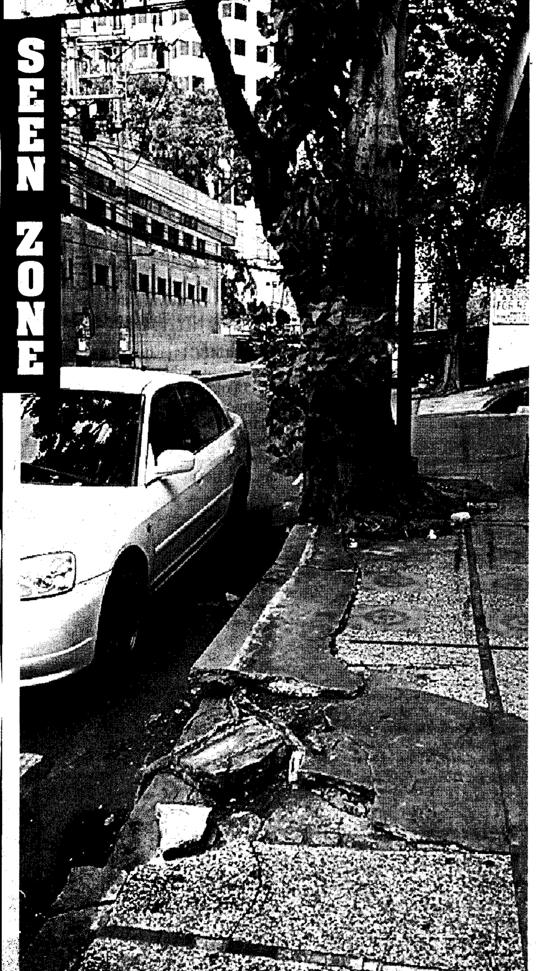
SIDEWALK REPAIR FAILS — The roots of this tree on M.H. del Pilar Street in Manila have broken through the sidewalk. Since it is illegal to cut trees, the local government tried to solve the problem by simply pouring concrete around it. The solution falled and the sidewalk is damaged again. (Carlo S. Suerte Felipe) #BeFullyInformed
